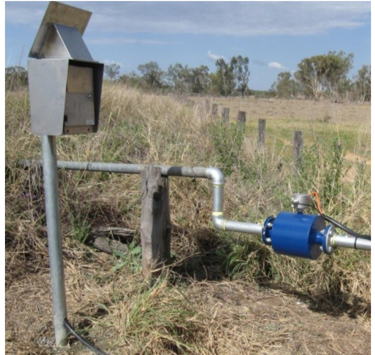
ENVOY station providing remote monitoring of a Pentair electromagnetic flow
